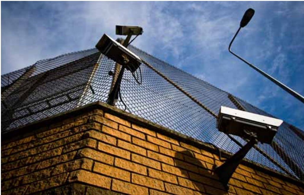
Police Service of Northern Ireland (PSNI) station at Grosvenor Road in the centre of Belfast. The fence is nearly ten meters tall and equipped with cameras to protect the Police against the attacks.
